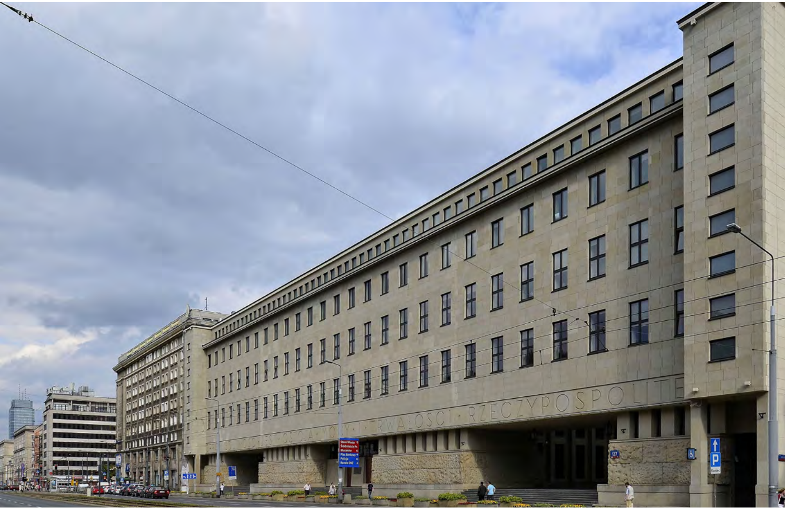
District Court in Warsaw [3]
